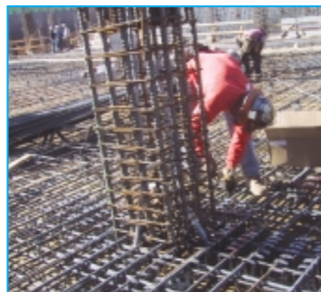
Shearband being installed
