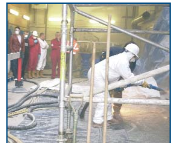
Course delegates watch a hands-on demonstration of concrete repair
